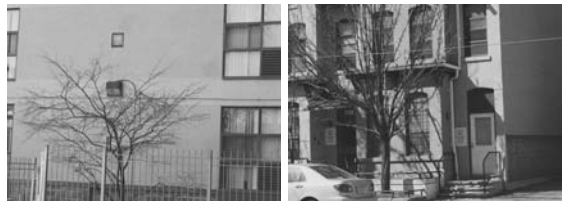
East end buildings after exterior stucco work
